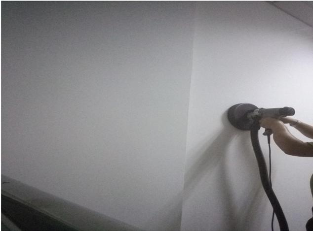
As shown on the picture the operator can sanding the different position of the wall.
