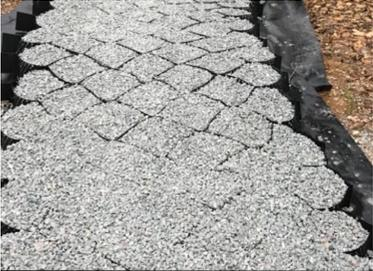
A photograph showing the geo grid installed on a prepared surface. The grid is covered with a layer of grey gravel, demonstrating the backfilling process. The grid's cells are clearly visible, and the gravel is being placed into them.                                                                                                                                                                           |
