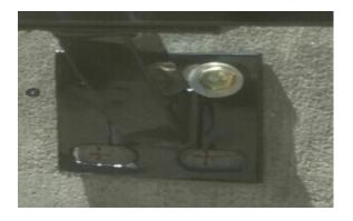
Step2: As shown, according to the installation position, fixed position, with a hammer drilling, the use of expansion screws will be fixed in the column base on the stairs.
